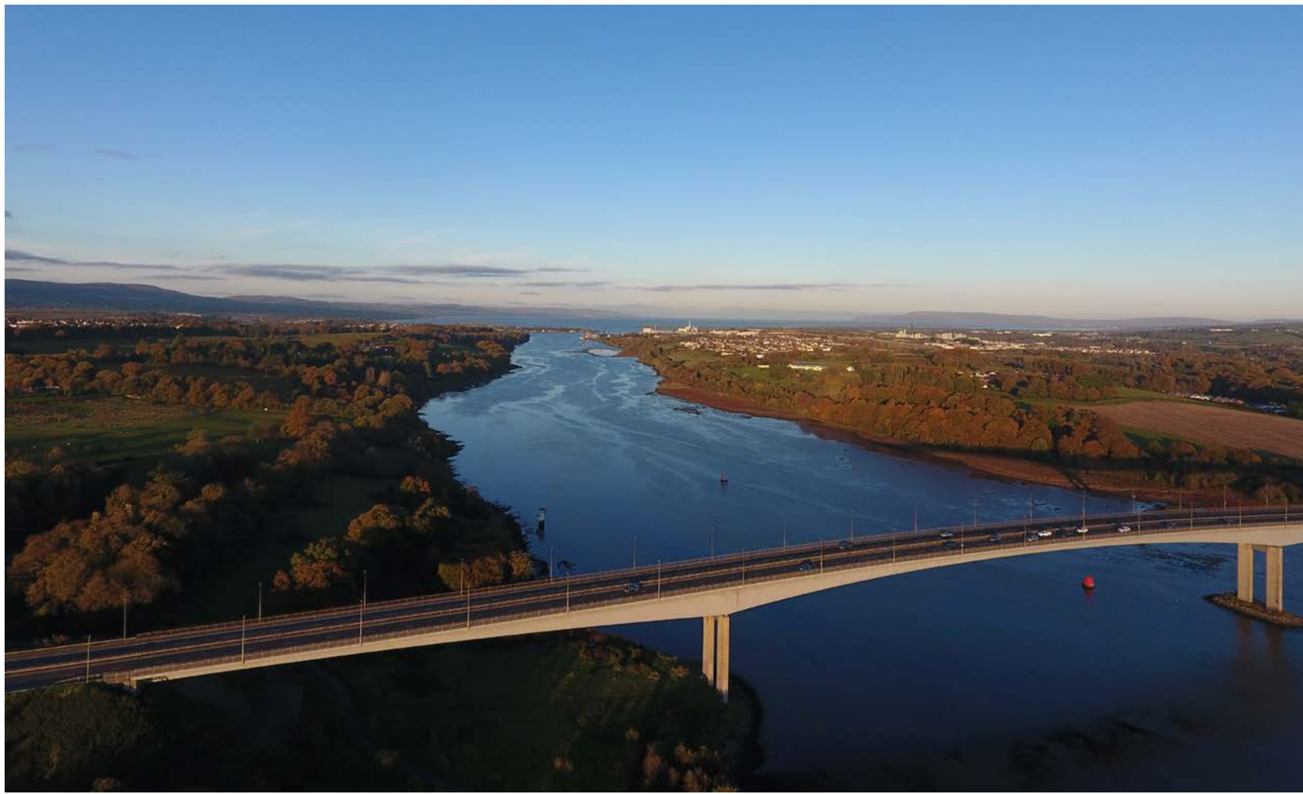
The proposed site is on the lefthand side of the photograph.
